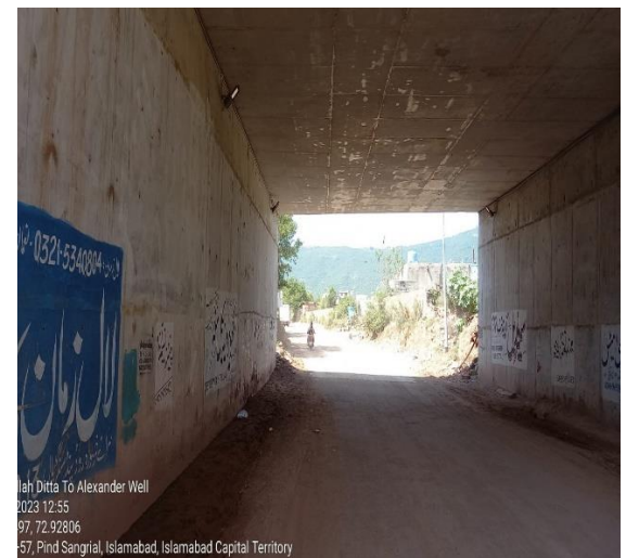
Exhibit 4: Shah Allah Ditta Underpass
