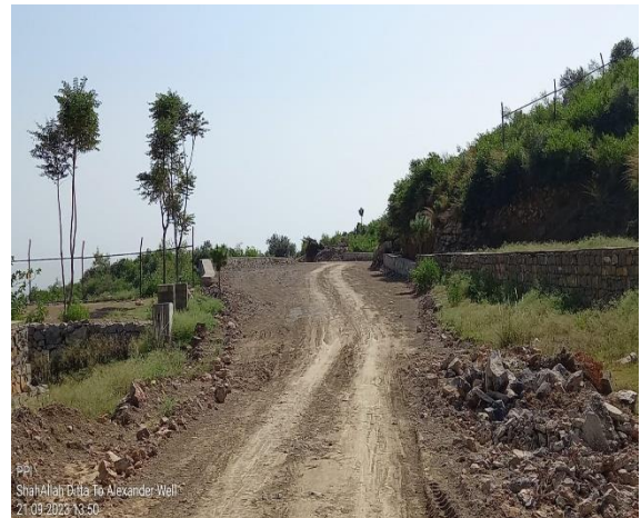
Exhibit 2: End Point of the project site
