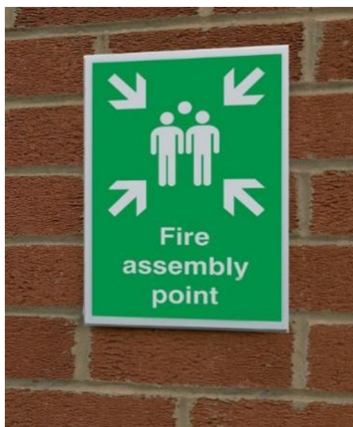
Figure 8.3: Typical Sign for Marking Assembly Point
