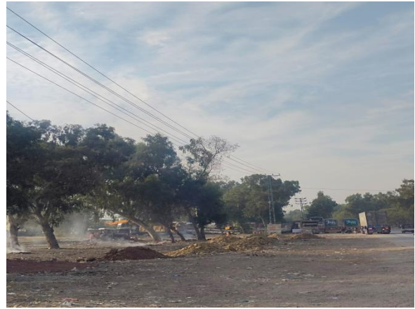
Exhibit 2: View of Peshawar-Rawalpindi Road (Access to project site)
