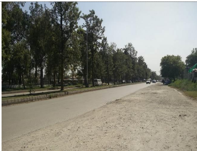
Exhibit 5.9: Ibn-e-Sina Road in the south of the project site
