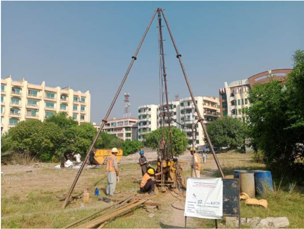
Fig 03: A view of site during performing SPT
