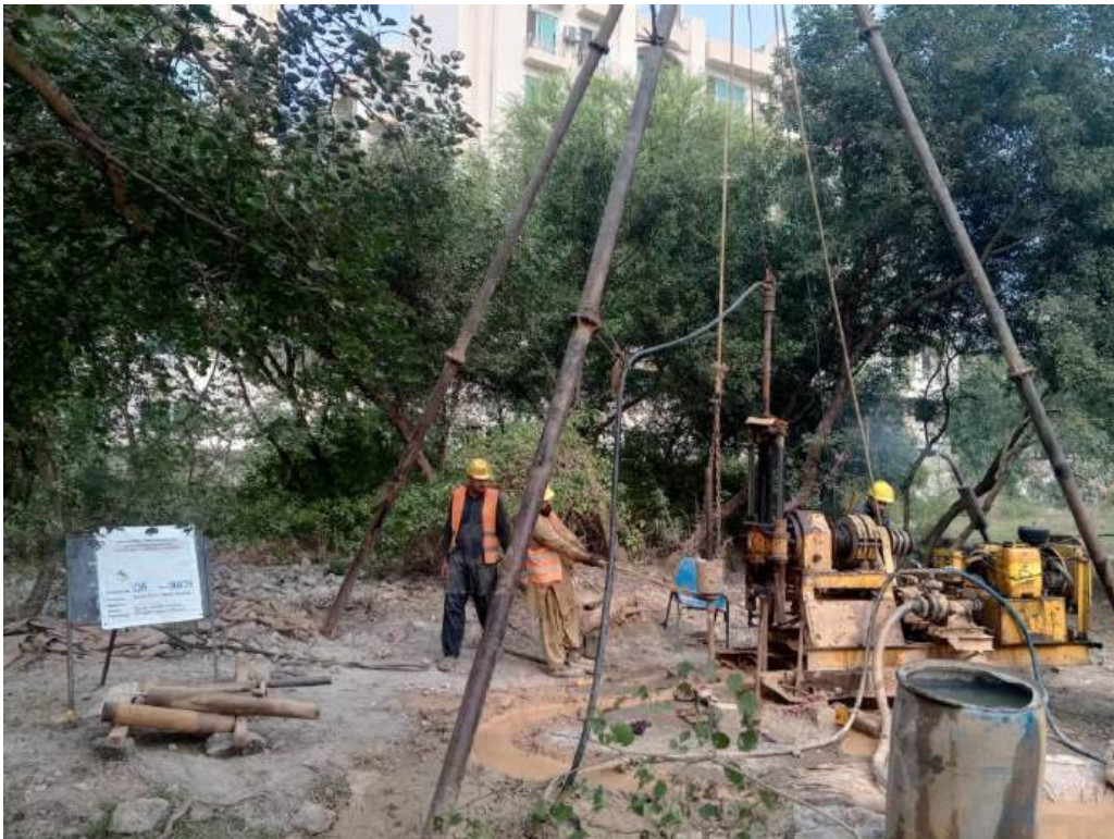
Fig 10: Another view of site during performing SPT
