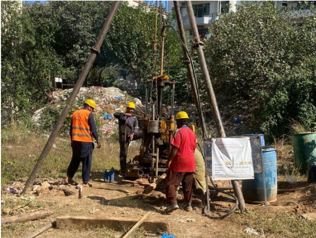
Fig 07: A view Drilling Operation at Site
