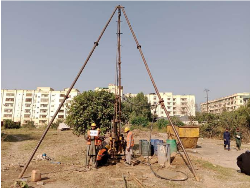
Fig 01: A view of site during performing SPT
