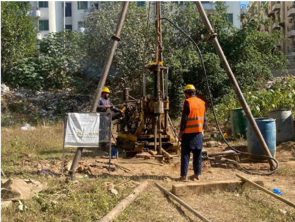
Fig 08: Another view of site during performing SPT
