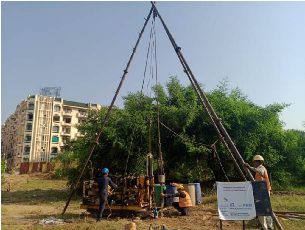
Fig 04: Another view of site during performing SPT
