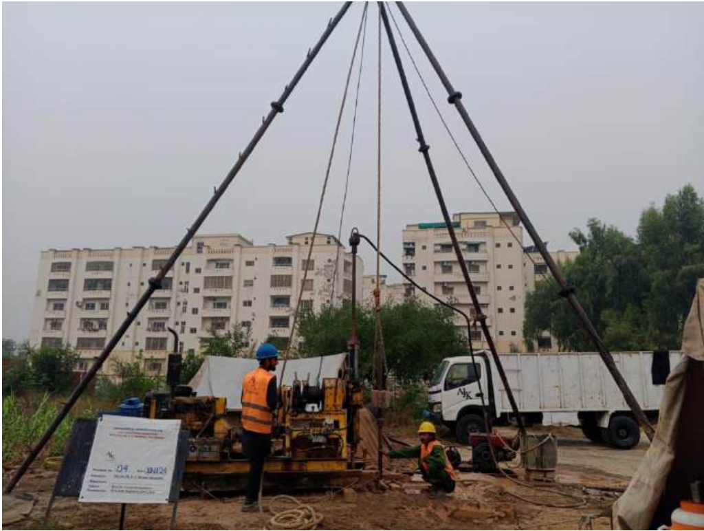
Fig 05: A view of site during performing SPT
