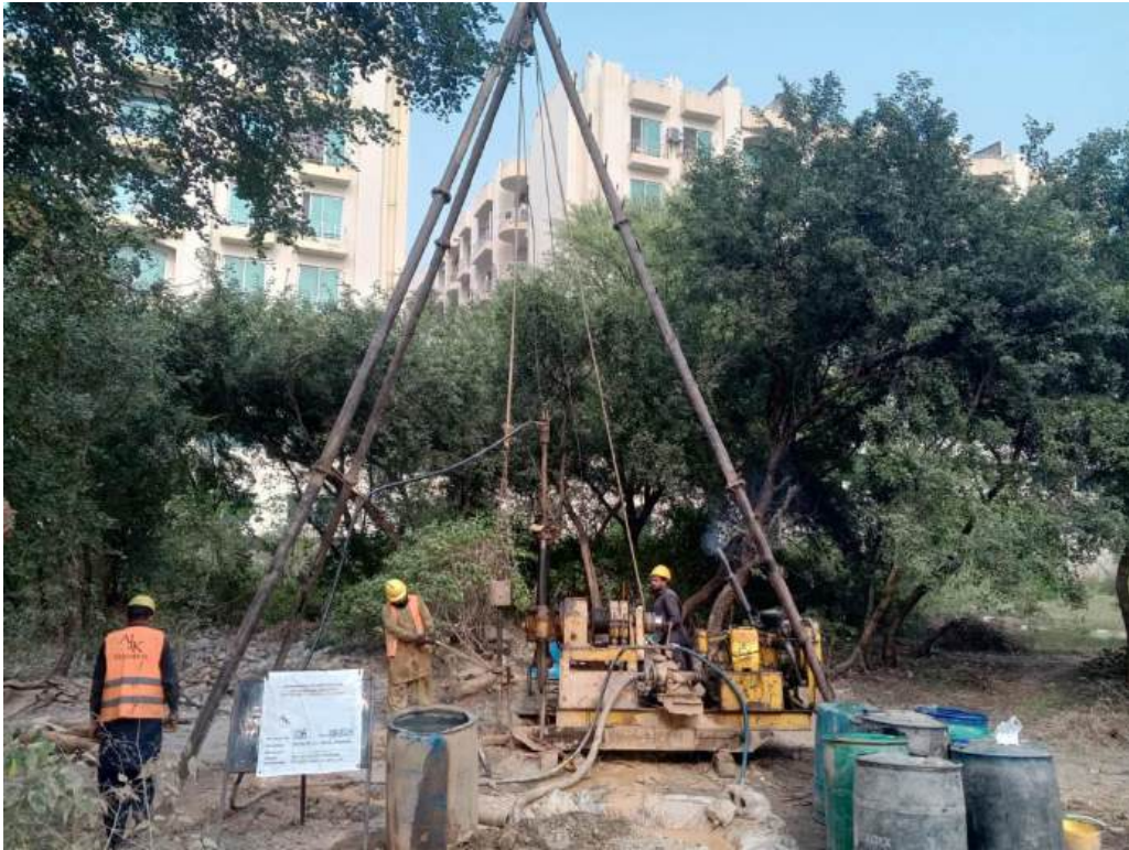
Fig 09: A view of site during performing SPT
