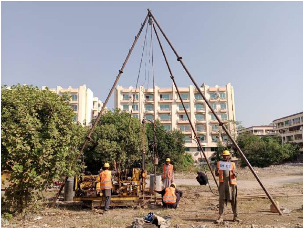
Fig 02: Another view of site during performing SPT
