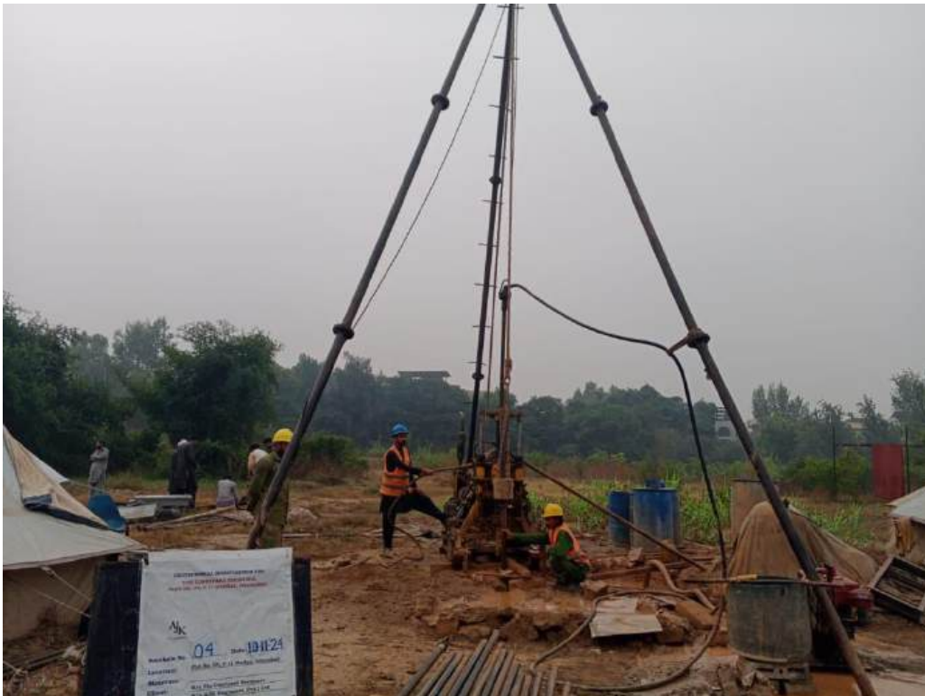
Fig 06: Another view of site during performing SPT
