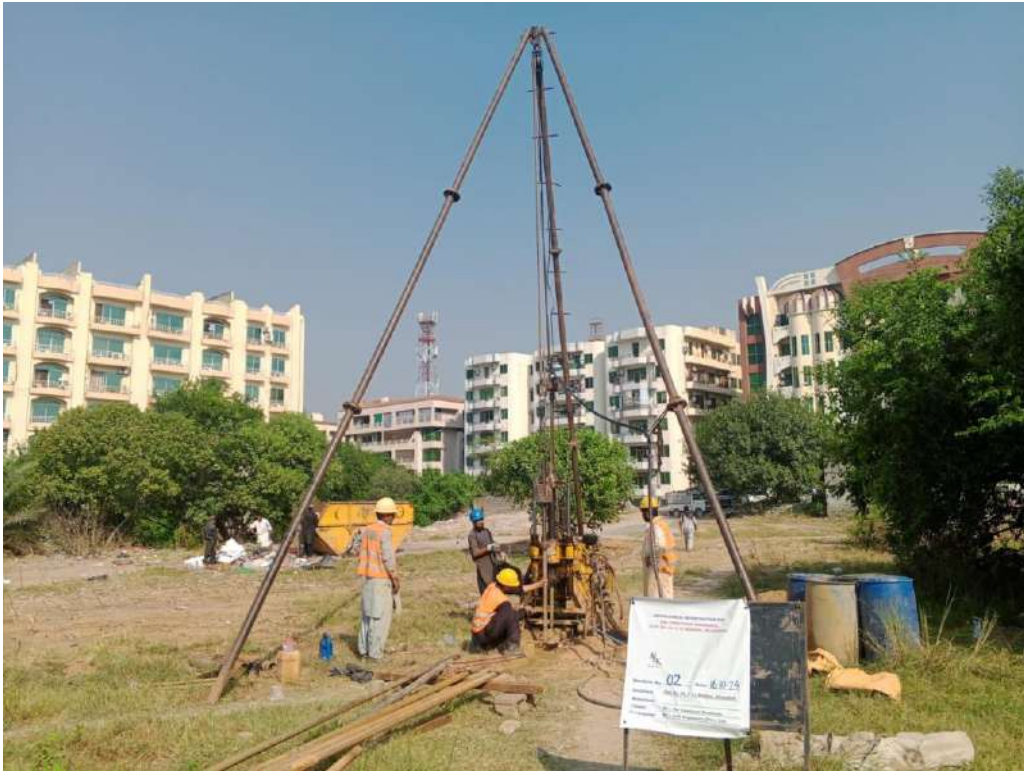
Fig 03: A view of site during performing SPT
