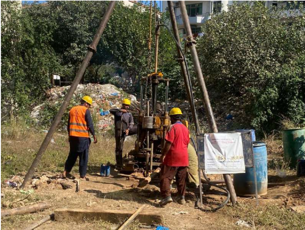
Fig 07: A view Drilling Operation at Site
