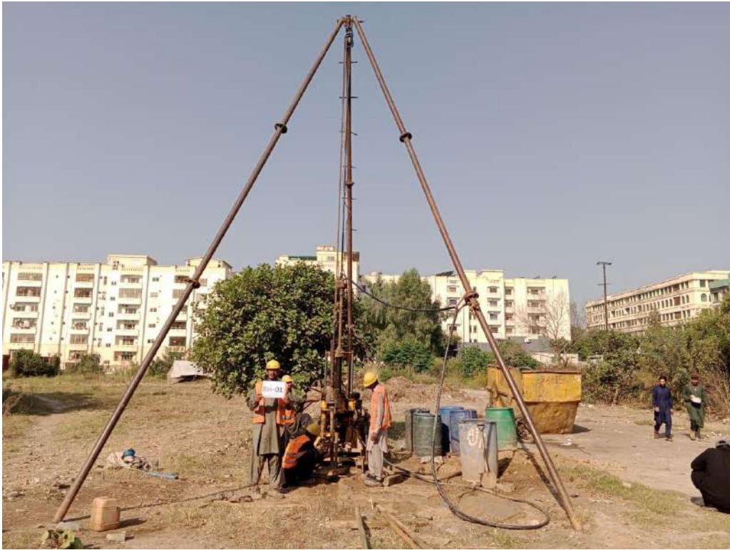
Fig 01: A view of site during performing SPT
