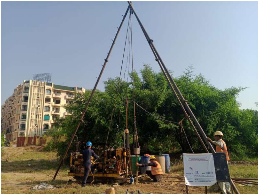
Fig 04: Another view of site during performing SPT
