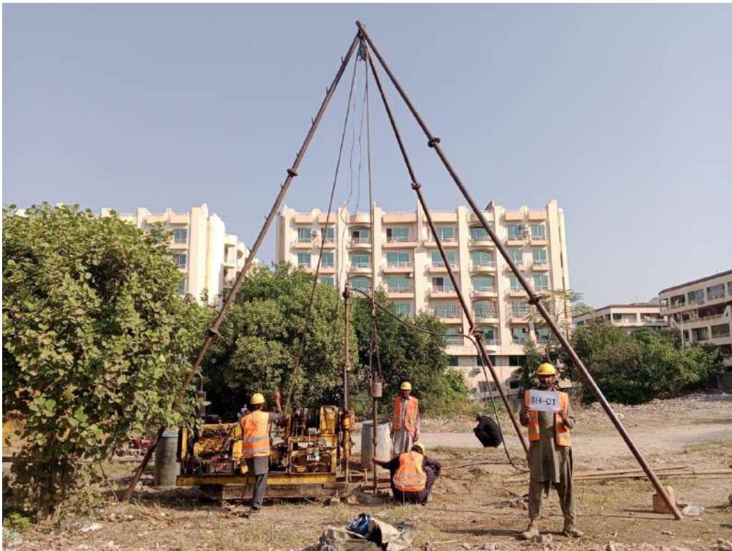
Fig 02: Another view of site during performing SPT
