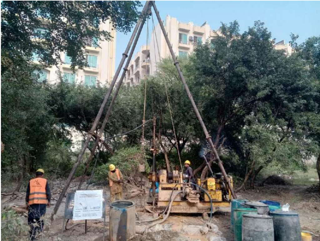
Fig 09: A view of site during performing SPT
