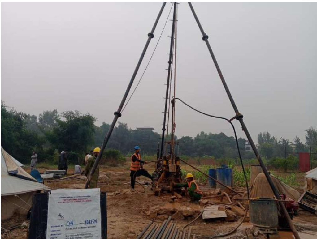
Fig 06: Another view of site during performing SPT
