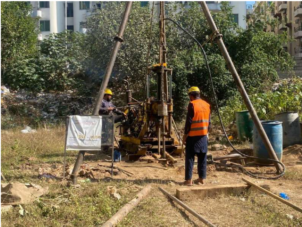
Fig 08: Another view of site during performing SPT
