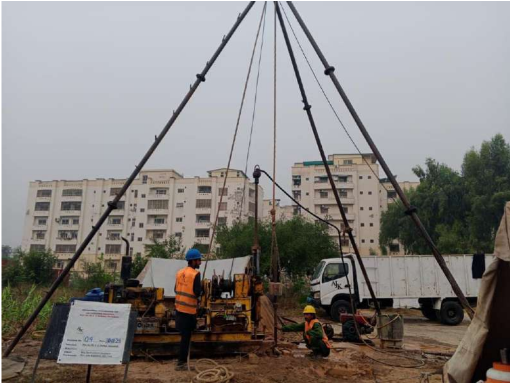
Fig 05: A view of site during performing SPT
