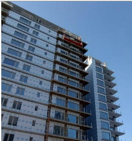
Exhibit 6.9: The underconstruction Sukh Chayn building near the project site
