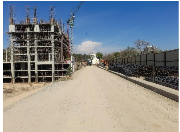
Exhibit 3.2: Access Road of the project
