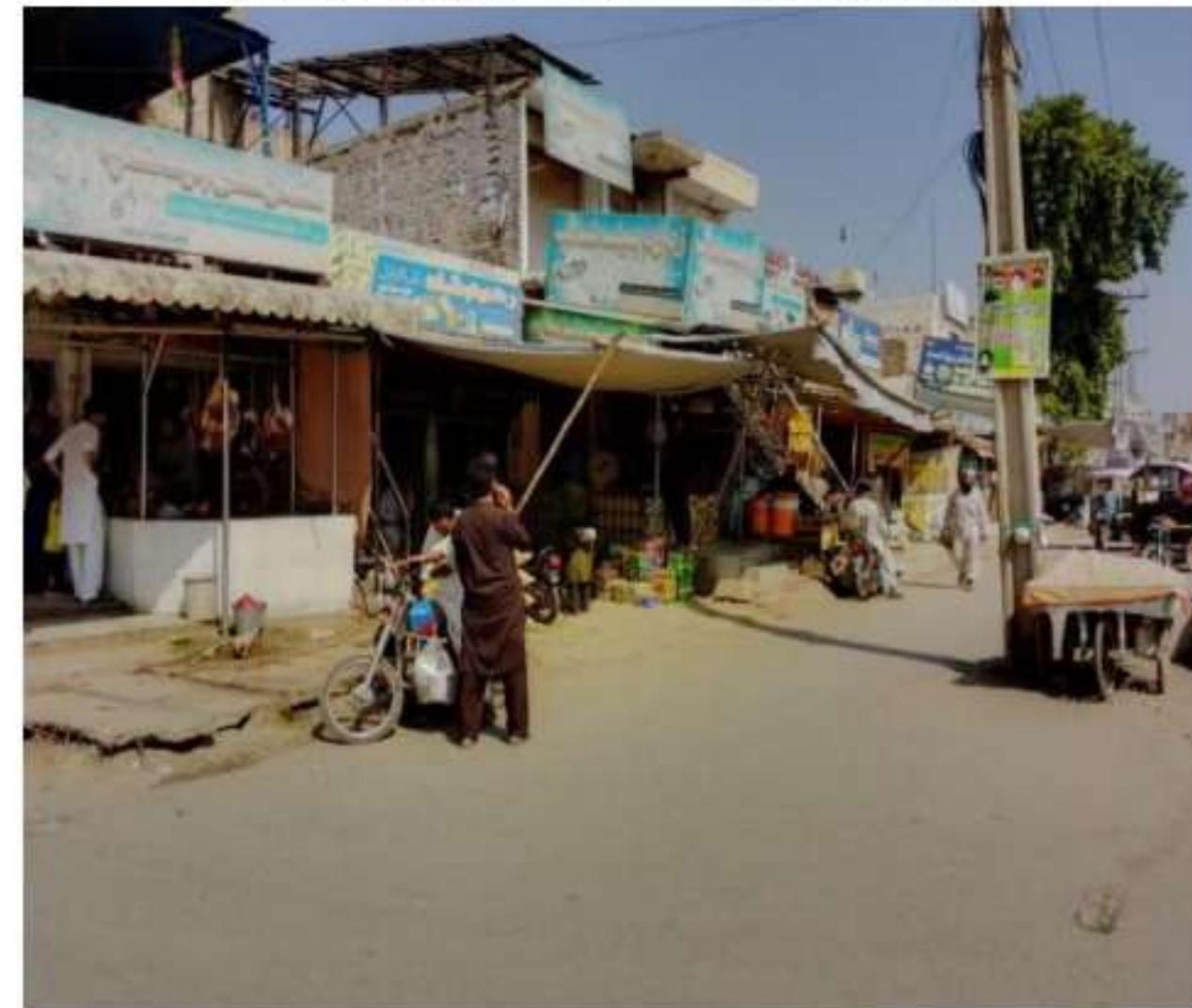
Shops within RoW of pabbi city (encroachment)
