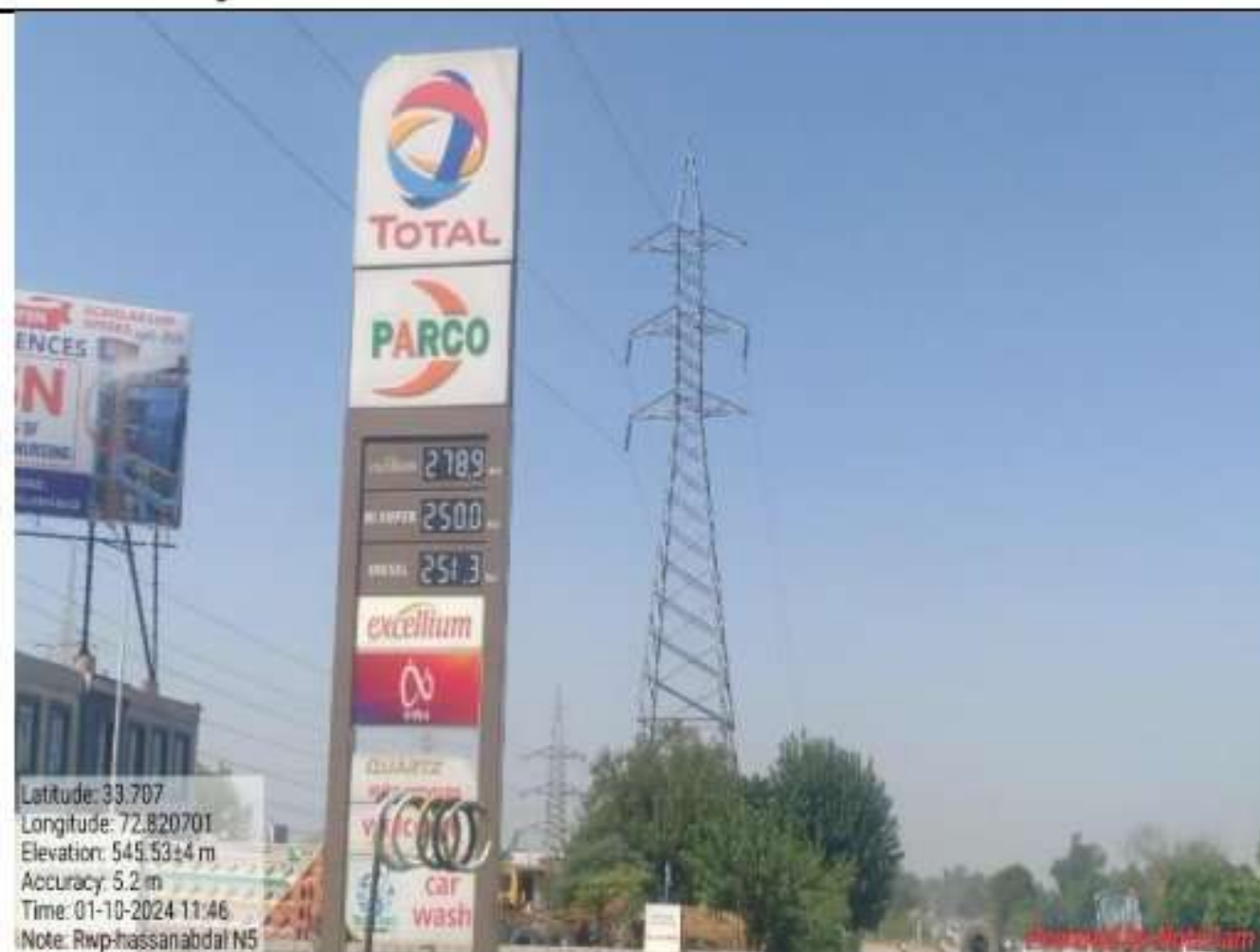
EHV Transmission Line crossings
