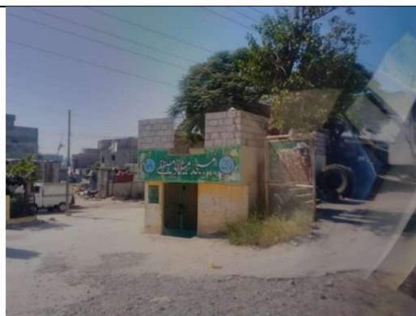
Mosque within row Wah Cantt. (encroachment)
