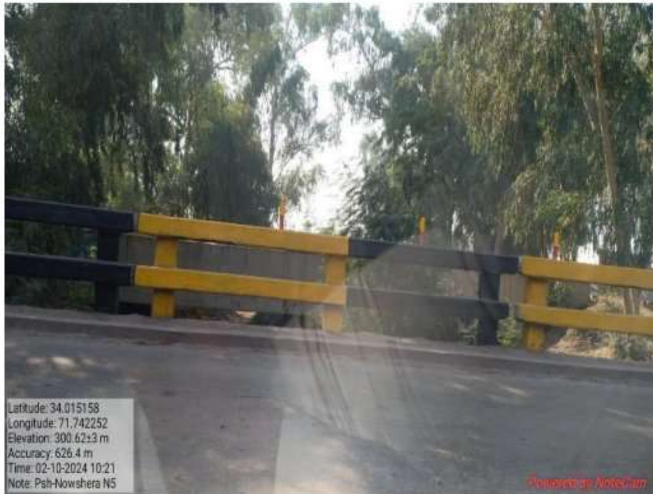
Bridge over Nullah
