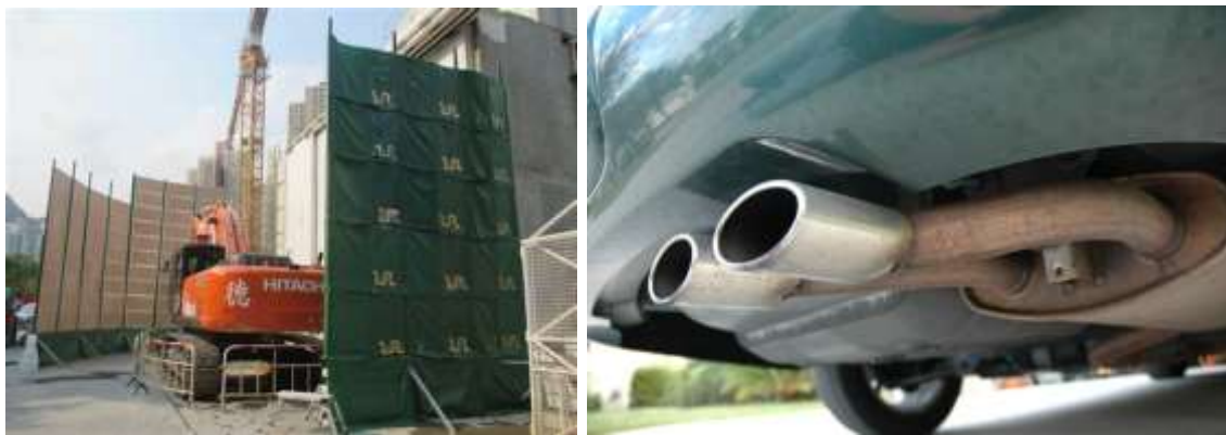
Figure 7.8: Noise Preventing Measures
