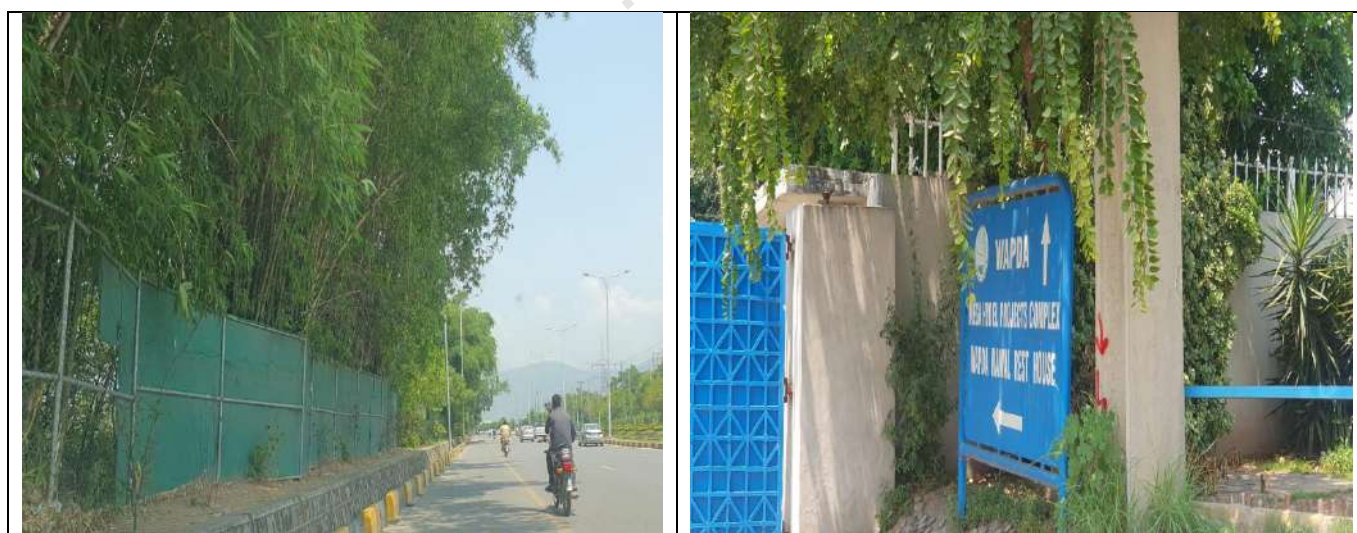
Figure 33: Structures more susceptible to damage during underpass construction and allied activities
