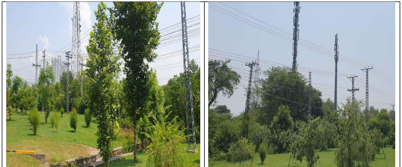
Figure 34: Traversing Overhead Utilities
