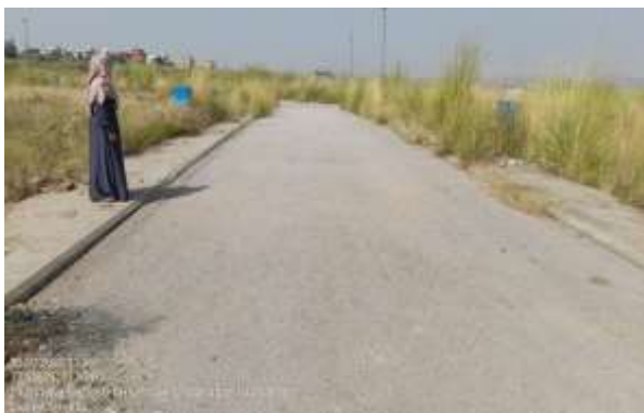
Exhibit 3.5: View of Streets Adjacent to the Project Site
