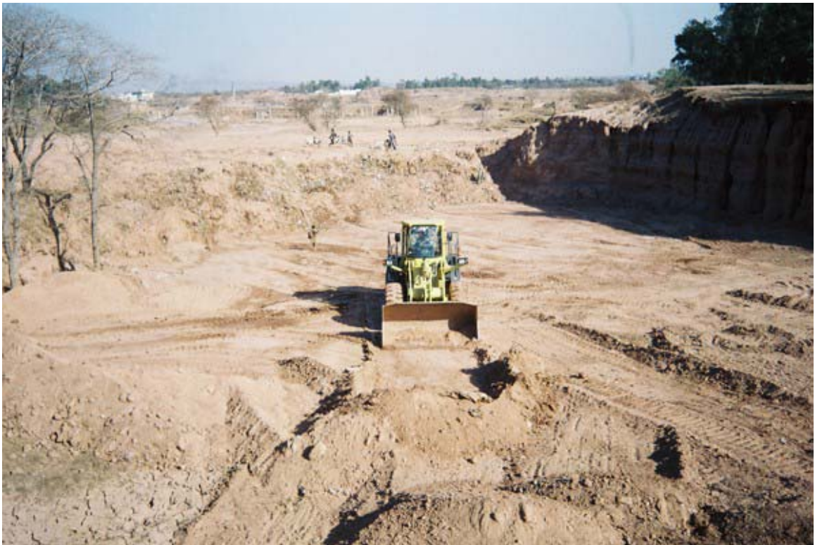
Figure 5.2-2 Landfill with daily cover soil
