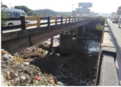
Bridge-2 @ Km 7+300 (Right Side)
