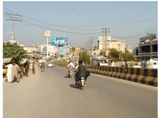
Bhaira Pul Bus Stop @ Km 9+000
