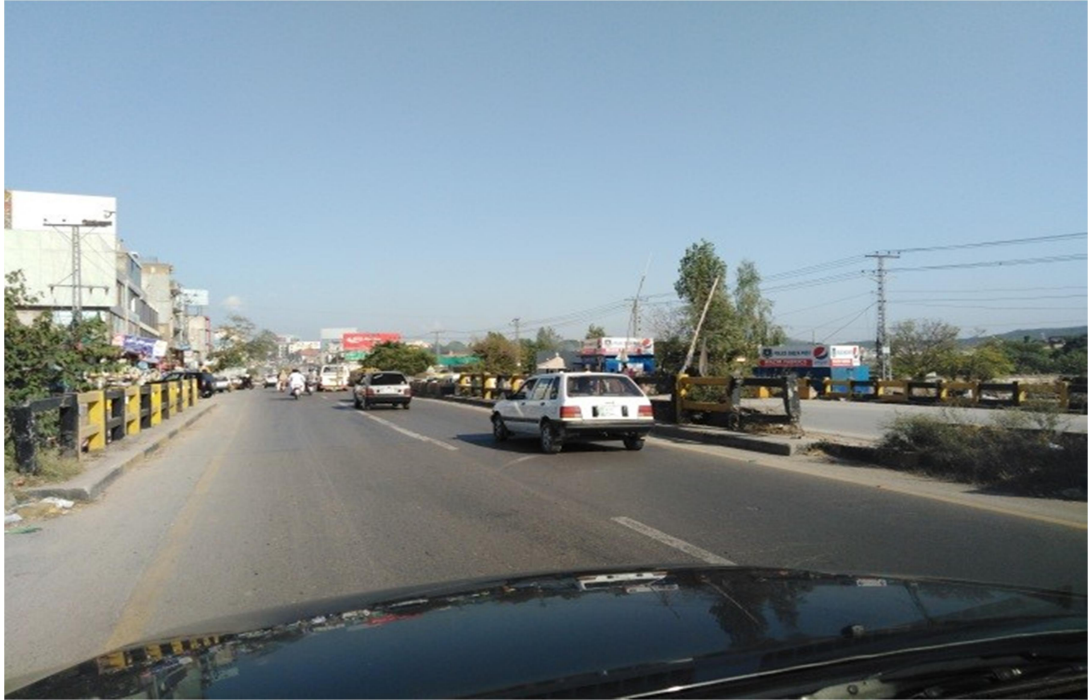
FIGURE – 4.9 : NULLAH BRIDGE NEAR JILLANI TOWN
