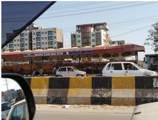
Bara - Kahu Bus Stop @ Km 8+500
