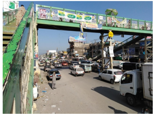
Pedestrian Overhead Bridge – Kiani Road
