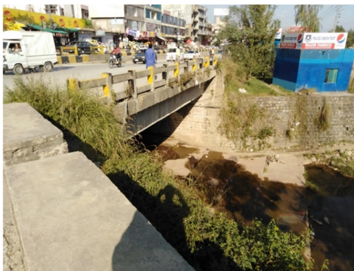
Bridge-1 @ Km. 6+800 (Right Side)
