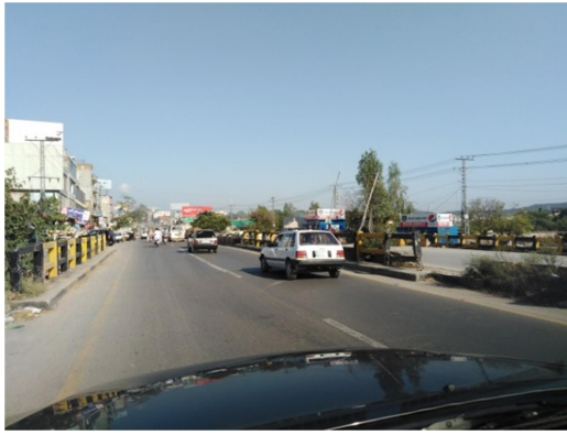
Nullah Bridge near Jillani Town
