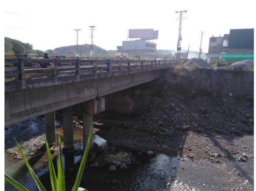
Bridge-2 @ Km. 7+300 (Left Side)
